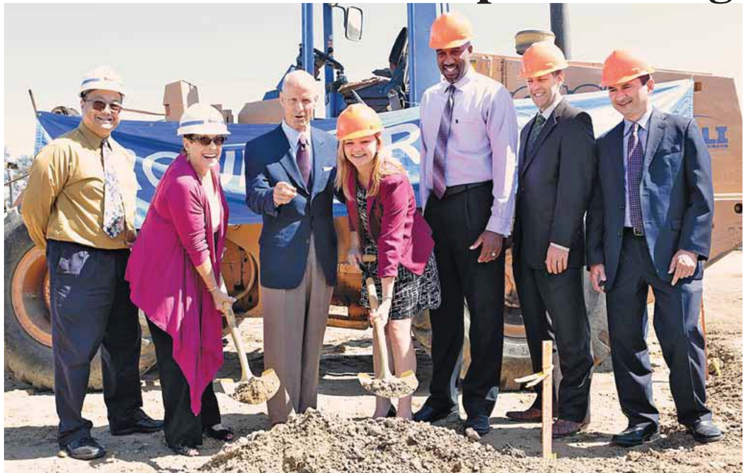
El Camino College celebrated the groundbreaking of a new Shops Building. The Shops Building will be a brand new 44,400-square-foot, state-of-the-art learning center, complete with indoor and outdoor learning spaces. The $31.8 million project is made possible with funds from the college's 2002 Measure E facilities bond. The new Shops Building replaces one of the first structures built on campus, dating back to 1949. Pictured is ECC Superintendent/President Thomas Fallo (center) with El Camino Community College District Board members (l to r) Ray Gen, Mary Combs, Brooke Matson (student trustee), and Ken Brown. Also pictured at right: Citizens' Bond Oversight Committee members Kirk Retz (committee chairman) and Nilo Michelin (committee member and Hawthorne councilman). Photo courtesy of El Camino College.
